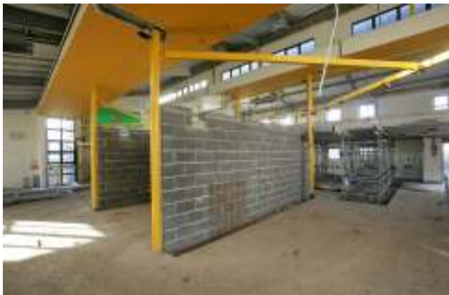
(Work to Technology Block is Underway)
